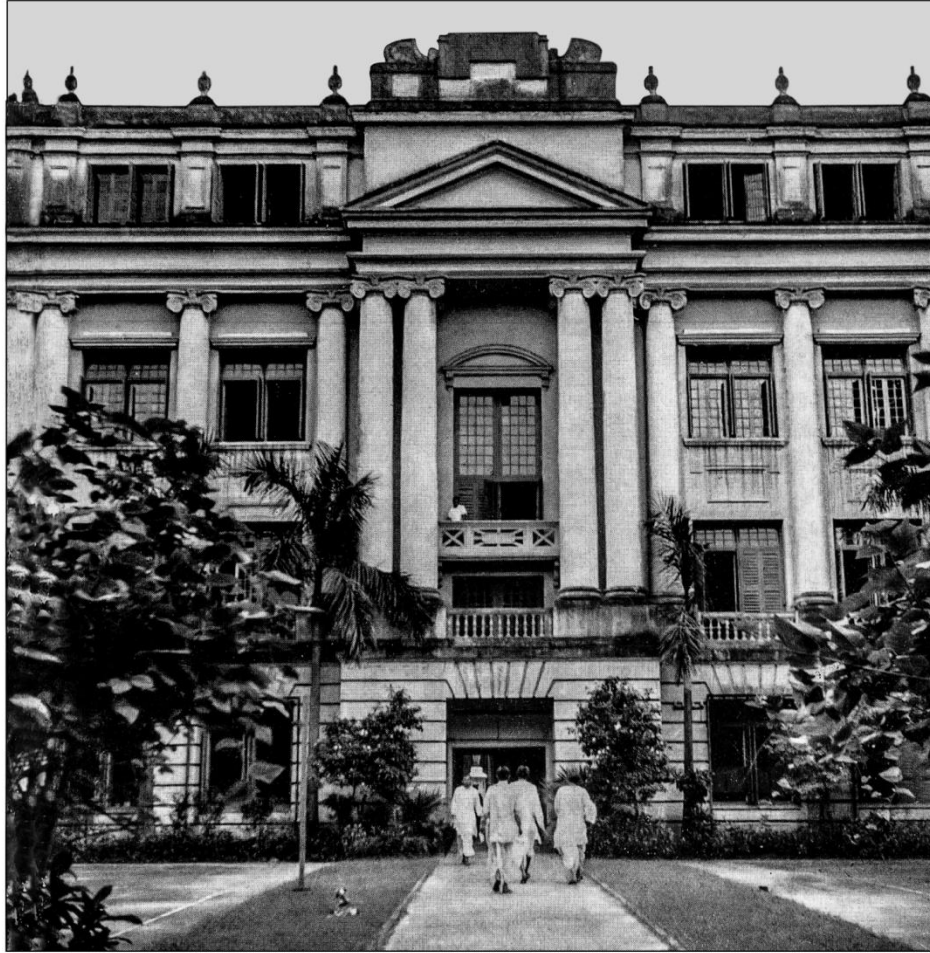
The Asutosh Building which is the seat of the College of Arts, the College of Commerce and the Central Library
